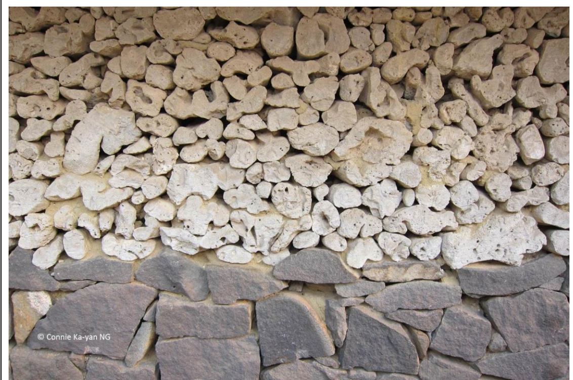
Picture 22. Local people use dead coral skeleton to build houses at Xuwen, Zhanjiang 圖 22. 在湛江徐聞當地人用已死的珊瑚骨骼建房
