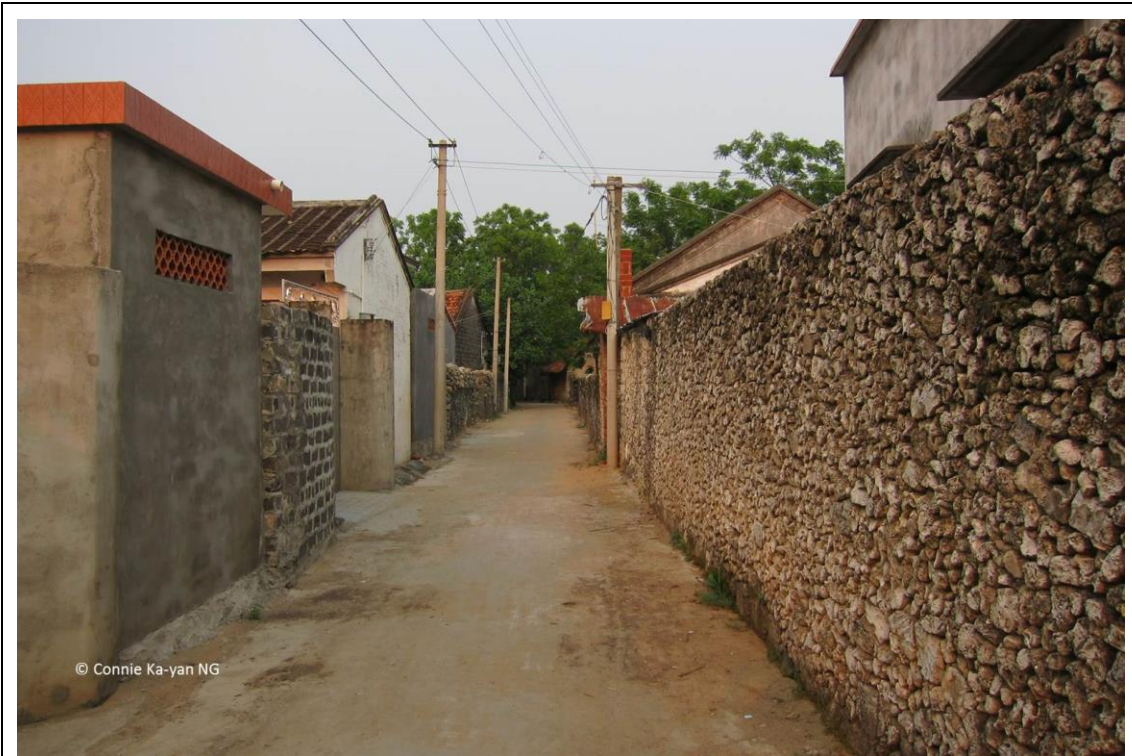
Picture 21. Local people use dead coral skeleton to build houses at Xuwen, Zhanjiang 圖 21. 在湛江徐聞當地人用已死的珊瑚骨骼建房
