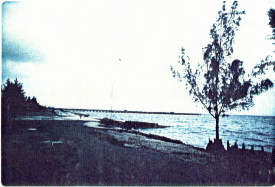
Plate 21. Midway Lagoon. Small boat launching ramps are in the center foreground and two 1,000-ft concrete piers are in the background.
