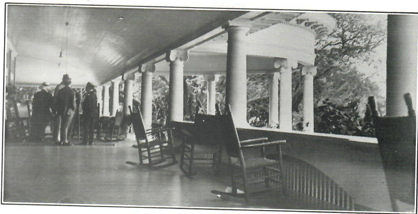
PORCH OF THE HALEIWA HOTEL.
