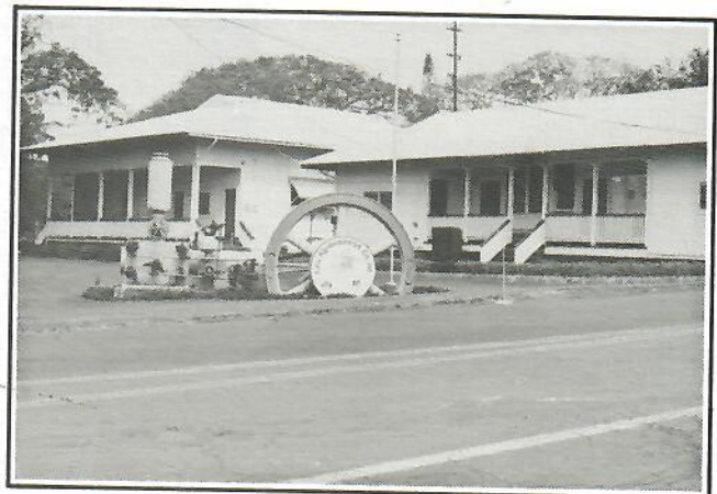
KA'U AGRIBUSINESS OFFICES IN PAHALA TODAY.
