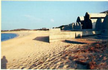
The construction of bathroom-toilet combination not only increase the beach erosion, but block the entrance of the tourists to the beach, results in more beach erosion.
