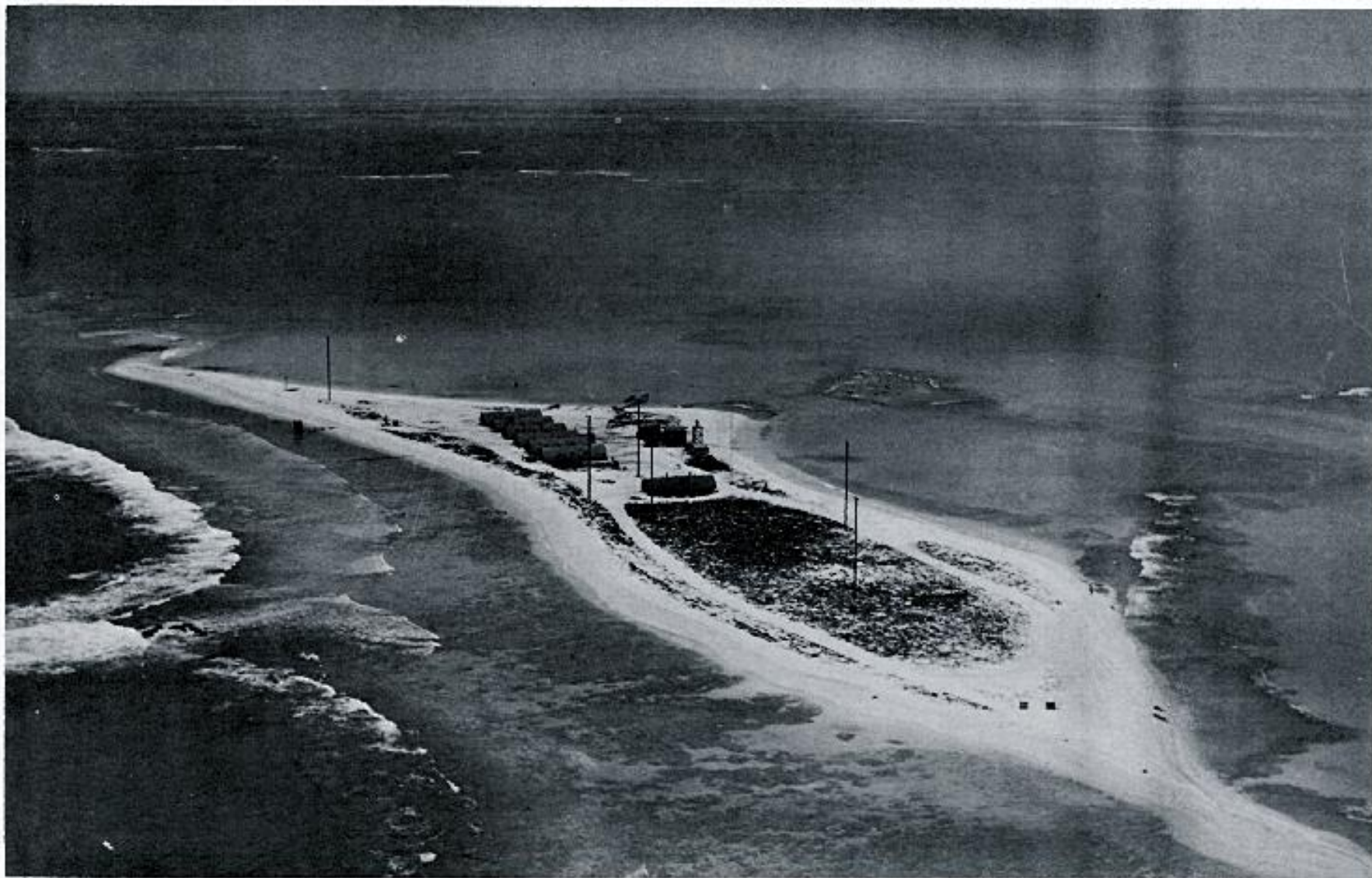
Figure 34. Newly constructed East Island Coast Guard LORAN Station, 24 April 1945. Official U. S. Navy photograph.
