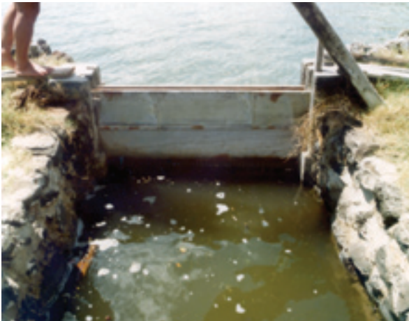
FIGURE 26: 'ĀUWAI SHOWING WEIR OR MOVABLE GATE SYSTEM
