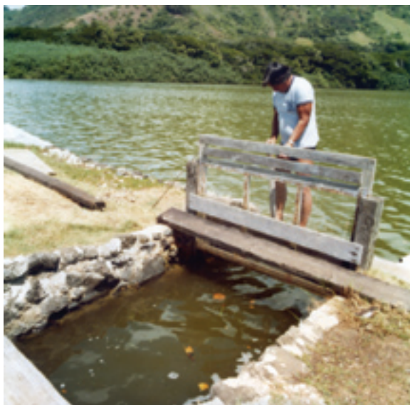
FIGURE 23: A SCREEN MESH ON TOP OF THE WEIR BOARDS FILTERS WATER DURING HIGH TIDES.
