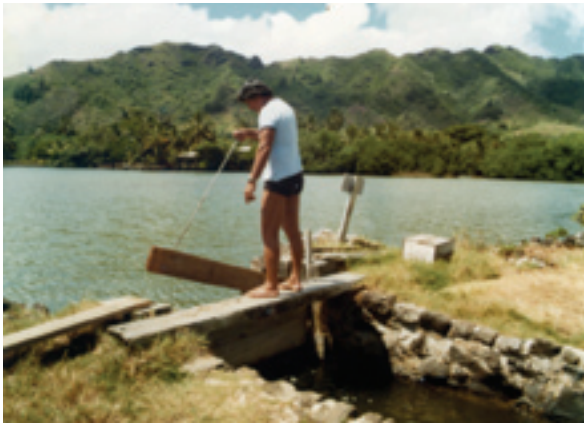
FIGURE 25: LIFTING THE GATE
