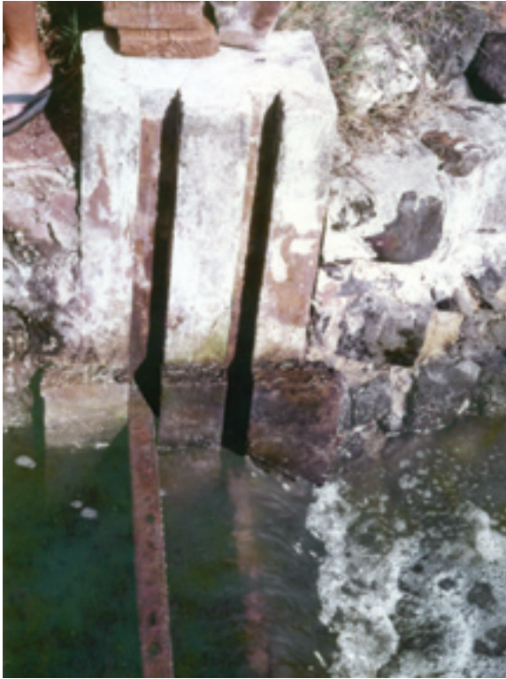
FIGURE 27: CLOSE-UP SHOWING GROOVES FOR BOARDS
