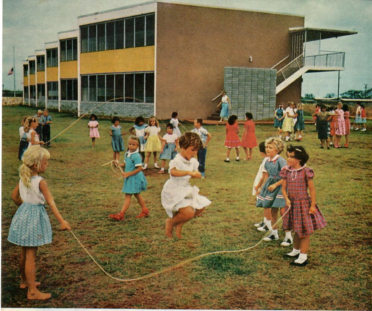
"Lady, lady, turn around. . . ." Rope twirlers chant the count at Oahu's Ewa Beach Elementary School. Glass walls and open-air corridors of the modern building take advantage of Hawaii's bright, pleasant weather. Flag flies at half-mast following Secretary Dulles's death.
