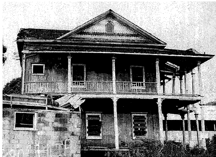
Figure 31. Wailuku Chee Kung Tong hall in 1988 with variegated shingles and arched vent at cross-gable similar to Waikapu hall. Decorative elements such as wood barge boards, roof combs, and dragons are removed. Courtesy Barbara Long.
