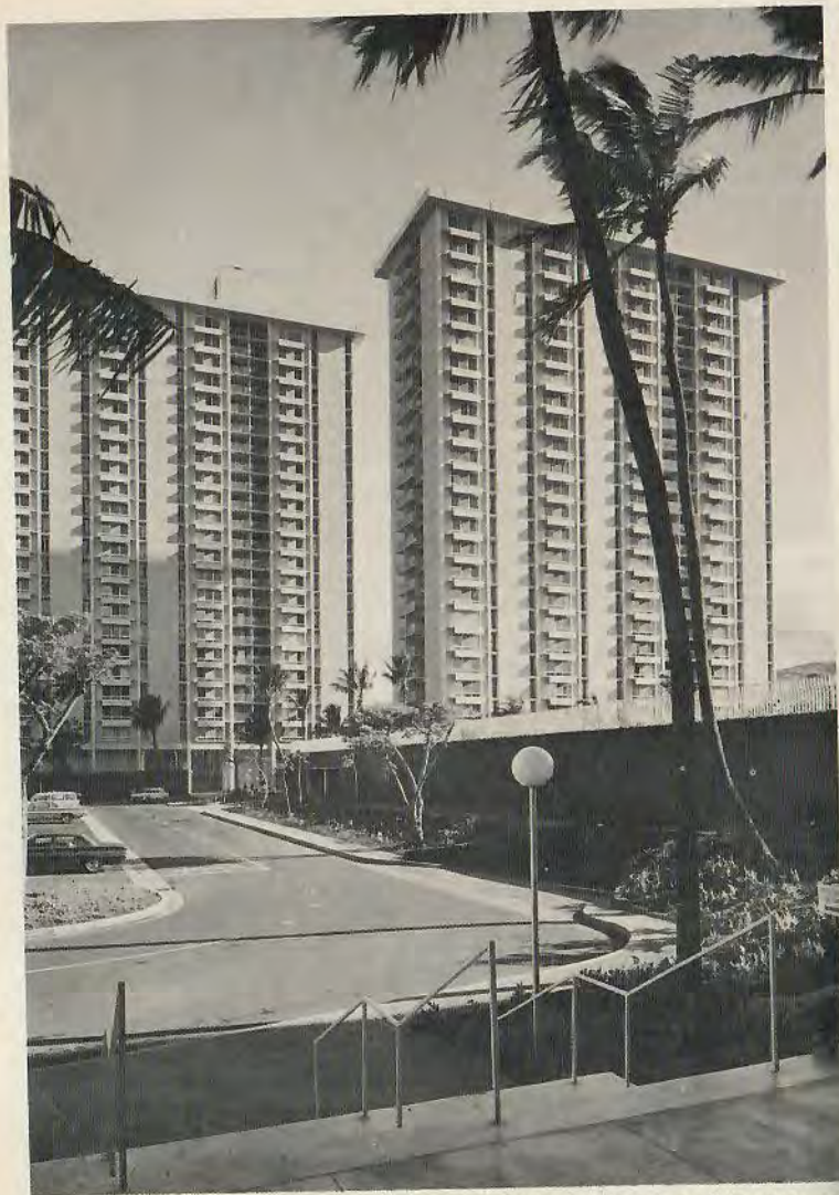
The Queen Emma Gardens adapts an international architecture to Hawaii's needs.
