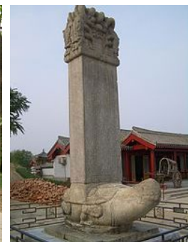
Stele in honor of the rebuilding of the Marco Polo Bridge by the
