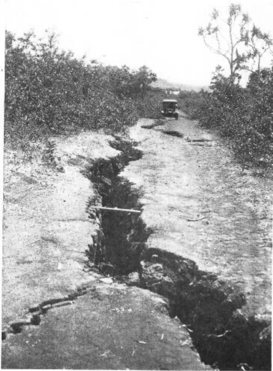
FIG. 2.—Cracks two feet wide, looking southwest toward Kapoho village. About April 24, 1924. Photo by Tai Sing Leo.
