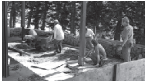
Workers repair the damaged lanai in front of the bookstore.
