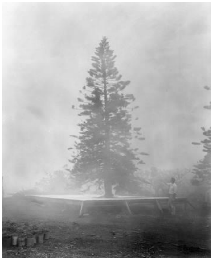
Fog Drip Station on Lāna‘i Hale – Cook Island Pine Catchment Platform. Up to 240 Gallons of Water Caught in 24 hours (1956).
