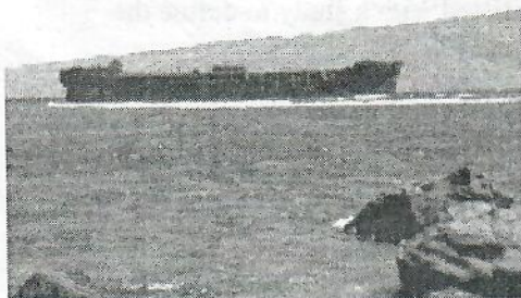
Unidentified ferro-cement wreck at Shipwreck beach, on the north coast of Lana'i. Photo by Hans Van Tilburg.
