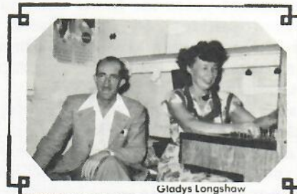
GLADYS LONGSHAW BASSETT at the Switchboard — 1947.
