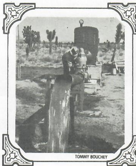
FLOWING WATER, at last. No more water hauling.
