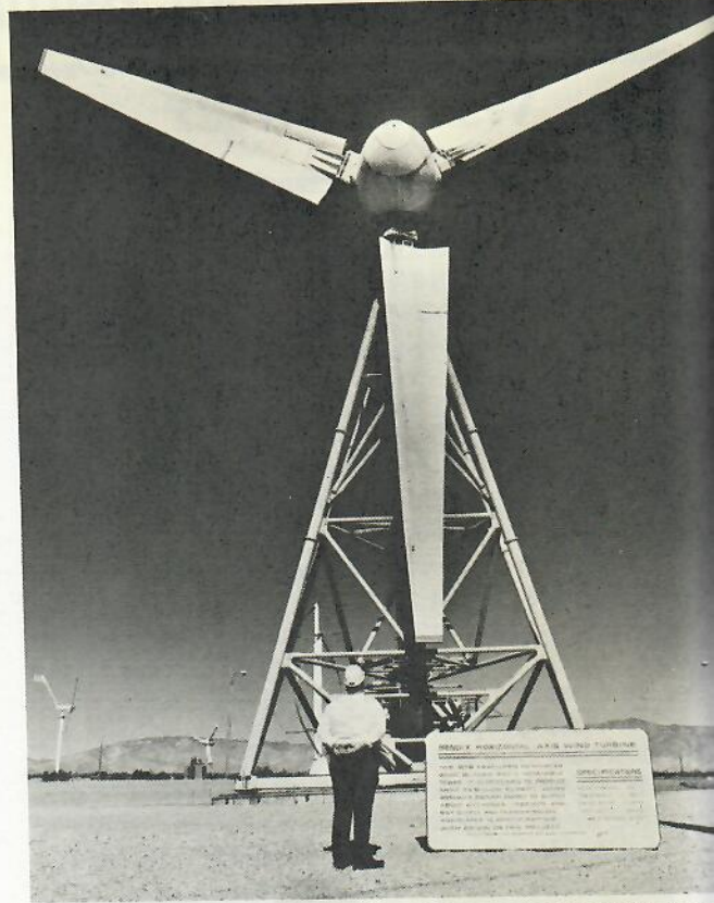
LANDMARK TURBINE COMPLETES TESTS — After nearly four years of operation, the Bendix Wind Generator (WTG) will be dismantled and removed from Southern California Edison Company's Wind Test Center, eight miles northwest of Palm Springs. The pioneer turbine began operation late in 1960. Experience gained is helping to improve design and reliability of newer WTGs.
