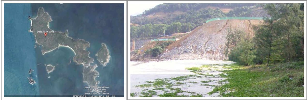
Plate 7 Left: Satellite image of Dalajia Island Right: Vocational facilities under the construction on the beach of Dalajia Island
