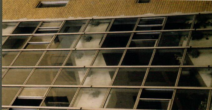
電信局東向柱幕牆 Detail of Glass Wall of Tainan Telephone and Communication Bureau
