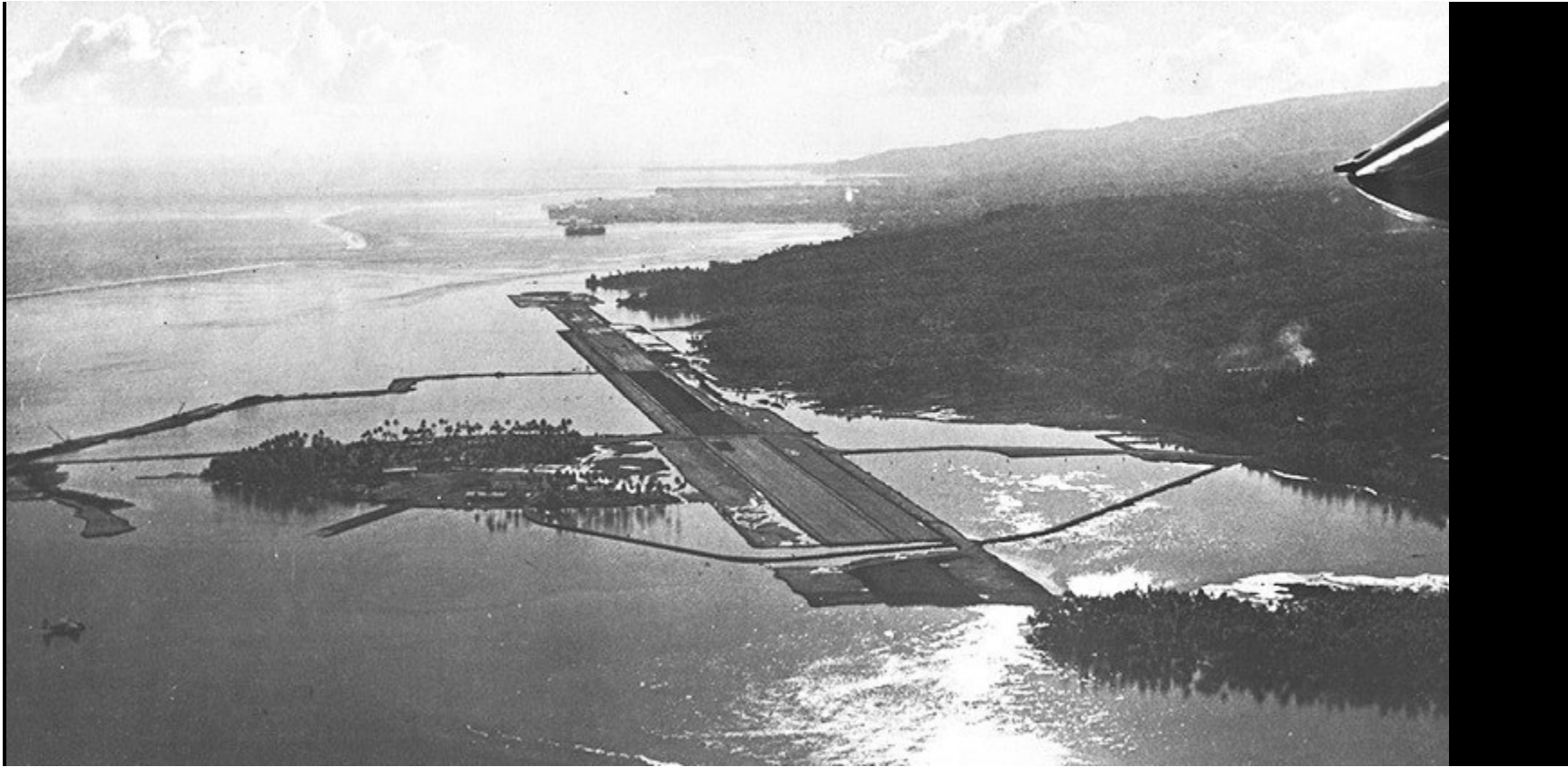
The construction of the Faa'a runway in 1960. It measured less than 2km on October 16, but reached 3400 meters a few months later, which allows it to accommodate jets.
