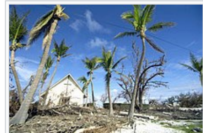
Damaged trees and debris left by Super Typhoon Ioke in 2006 at the Memorial Chapel on Wake Island
