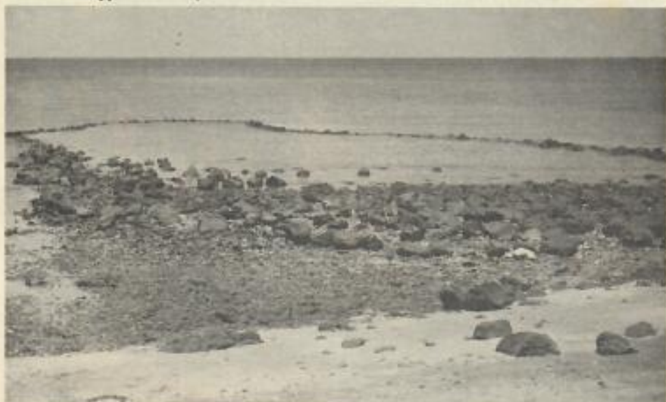
Fig.12. Stone fish weir, Darnley Island. These ancestral structures, which are still in use, not only help provide turtle feed but also may serve as models for construction of sea-crawls on the islands at which boulders are available.
