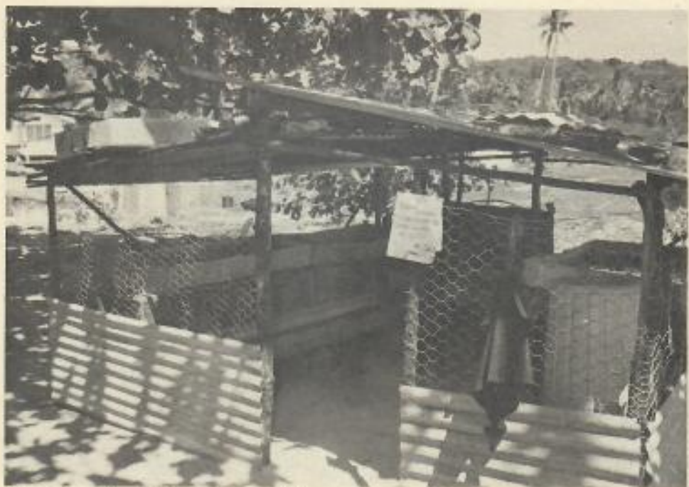
Fig. 6. Yam Island: farm of galvanized iron and poultry-wire construction and with tanks of galvanized iron.
