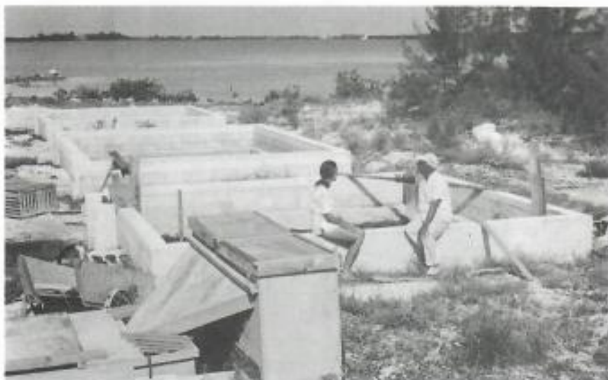
Looking west at our small turtle hatchery built by John M. Spottswood for my son and I to do our research about sea turtles. Notice the incubator and chute extending into the tank of seawater.
