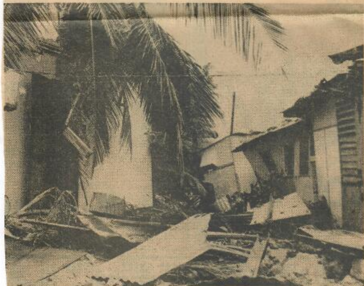
Some of the damage done by gale-force winds and 20-foot surf.
