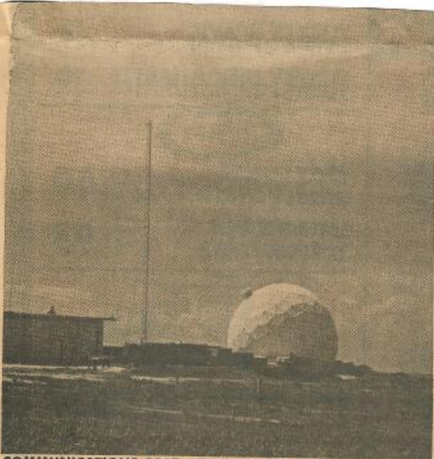
COMMUNICATIONS GEAR —The "golf ball" radome and antenna are part of the new military picture at Diego Garcia.
