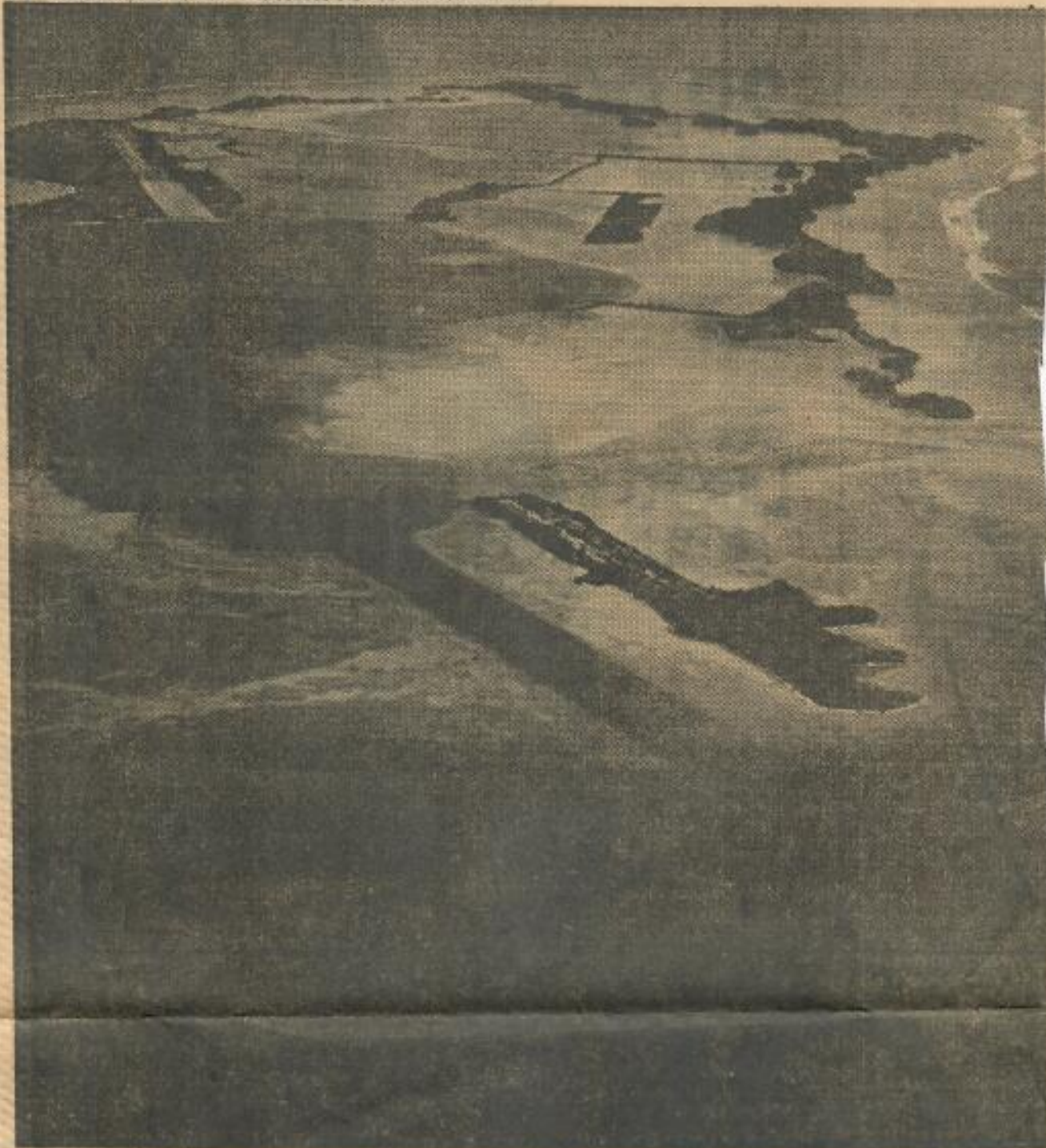
Palmyra from the air: Photo shows dredged channels and lagoon; causeways are built from dredged material.
