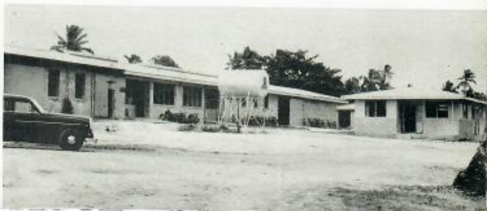
Niue's public works depot is an example of the islanders' ability as builders with concrete blocks.
