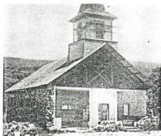
FIG. 6. West end of Pukaana Church at Hookena Beach showing complete demolition of masonry wall of this 100-year-old structure. Much of the debris was cleared away soon after the earthquake. No nearly comparable damage to this building is known to have taken place during the century since it was built.
