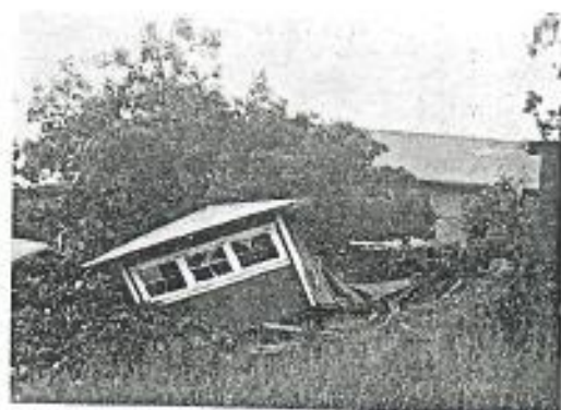
FIG. 4. Overthrown shop building at Kaimalino, from the south.
