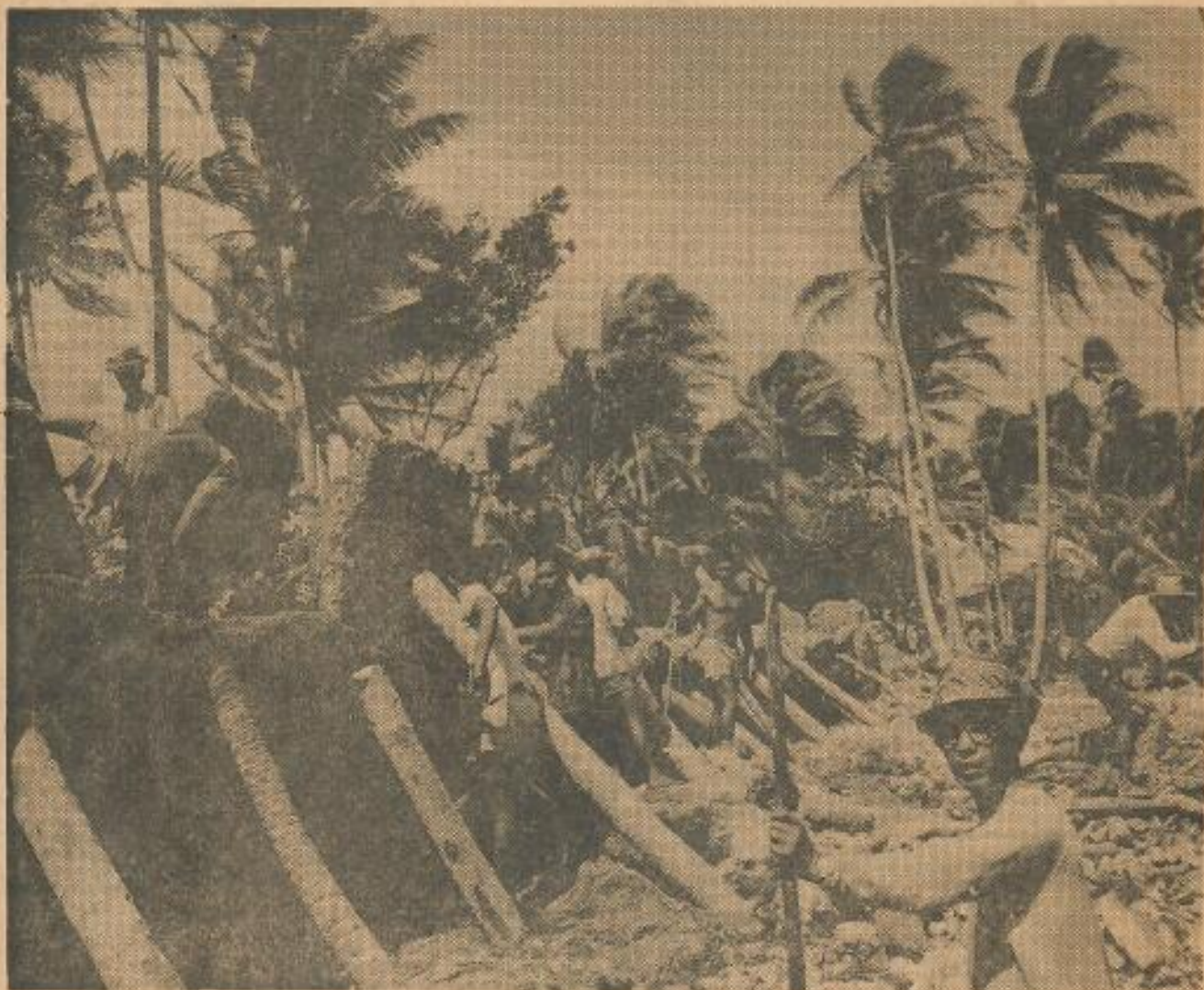
TOUGH JOB — Dr. Yoshihiko Sinoto, right, supervises the reconstruction of Marae Anini, national temple of Huahine Iiti in the Society Islands.
