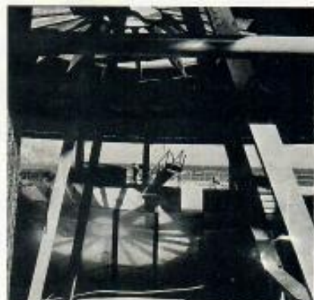
Ocean Science Theater under repair.
