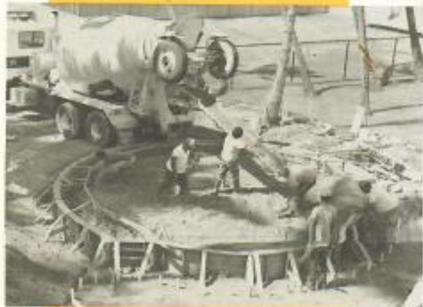
Pouring the foundation for the Hatchery tank...
