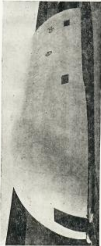
Figure 1.1. This portable warehouse is entirely supported by air. It is made of Fibertin, a paper-thin tough vinyl-coated nylon fabric produced by the coated fabrics department of U. S. Rubber at Mishawaka, Indiana. The structure is held to the ground by a tube at its base which is filled with water. A small blower keeps up the supporting air pressure, which is low. Passage through the door does not disturb the stability of the structure.
