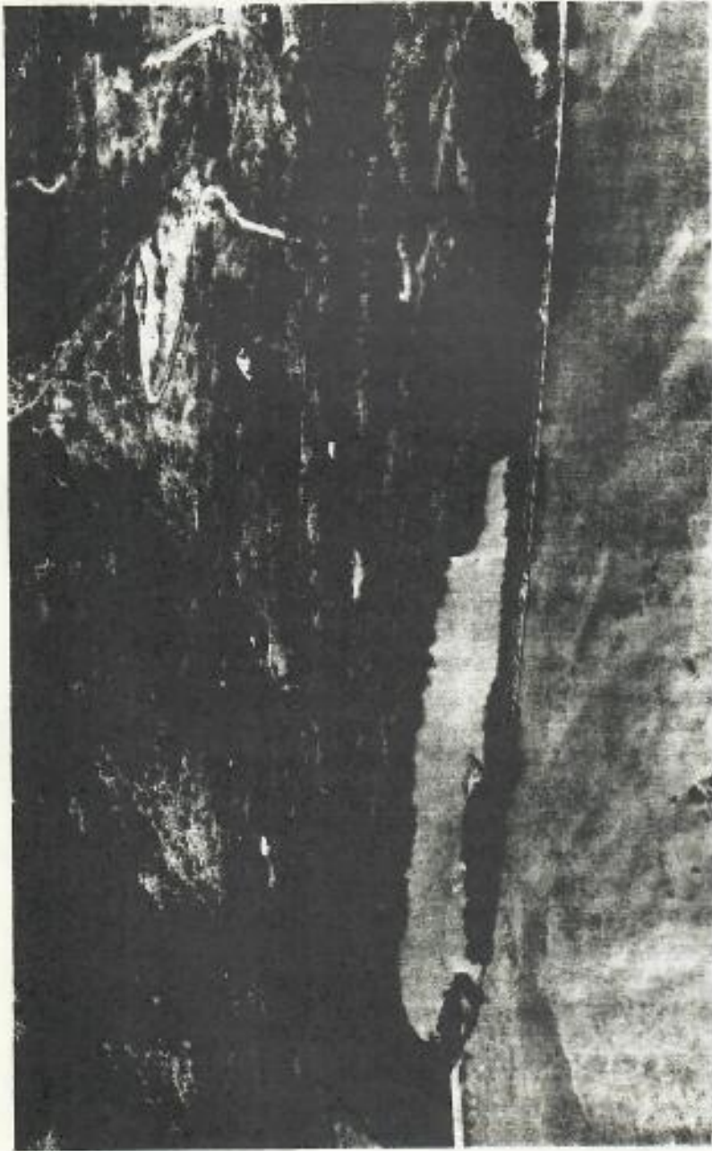
Figure 4. P'olip'o Fishpond, Molokai, shows the extent to which mangroves have invaded walls and colonized the sediments accumulated in the pond in the absence of periodic cleaning.
