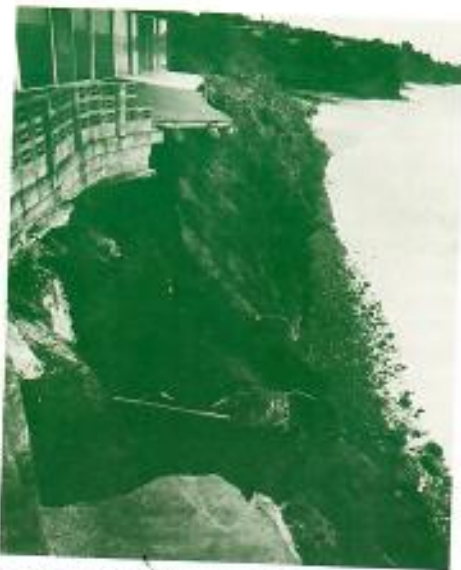
Ground failure caused by an earthquake.
