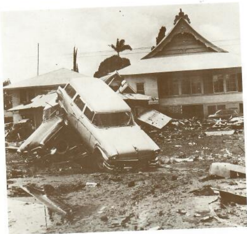
Damage caused by a tsunami.
