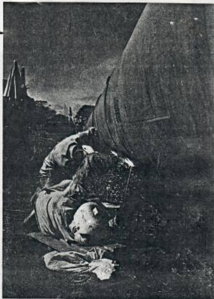
Pipe sections, 36 and 40 in. dia., are welded into double joints, transported to trenchside then bent, welded and placed.
