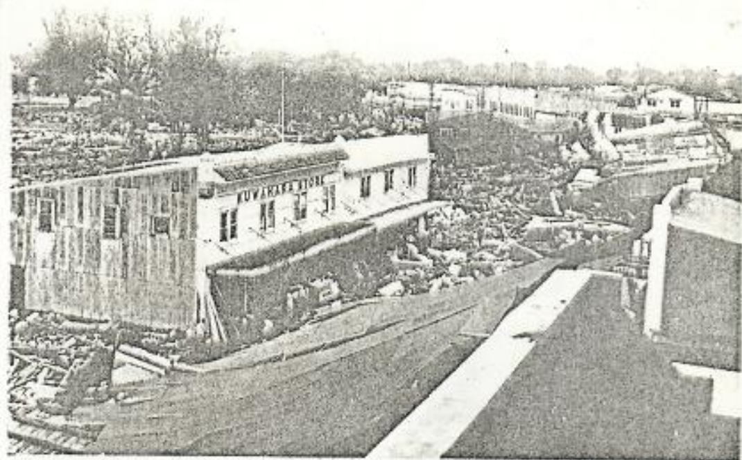
PLATE 3A. Wreckage left by the tsunami along Kamehameha Avenue, Hilo. Buildings on the left-hand (seaward) side of the street have been pushed into the street, some more or less intact, others as heaps of debris. Photo by Francis Lyman.
