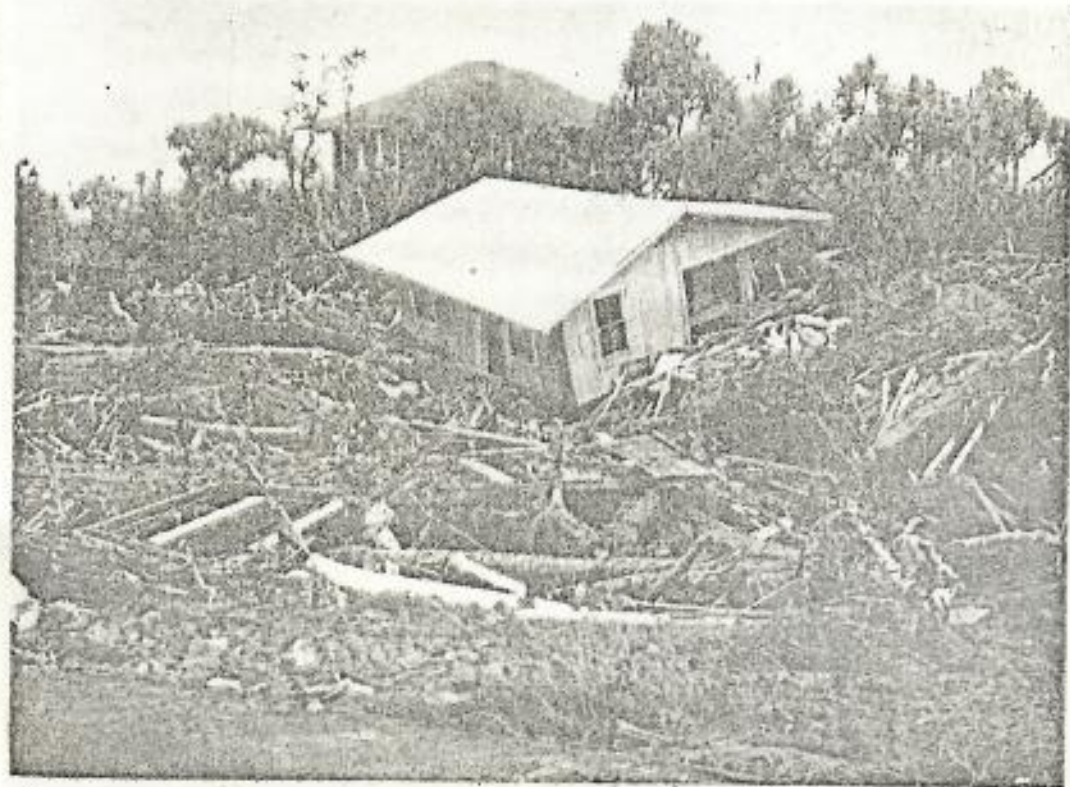
PLATE 3B. House in Keaukaha, east of Hilo, carried inland about 100 feet by the waves. The
