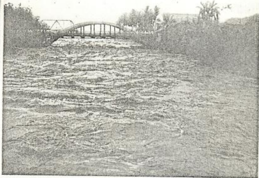
PLATE 5A. The very high stage of the water, in Wailuku River at Hilo, reached 3 or 4 minutes later than the stage shown in Plate 4B. Photo by Warren Flagg.
