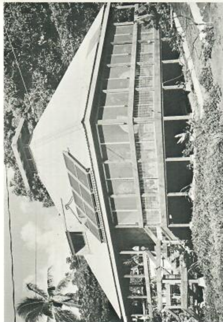
A rooftop solar water heater is among the energy saving devices at the University of Hawaii's energy house.
