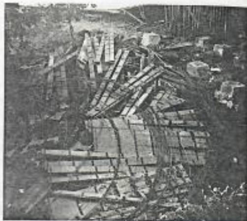
FIG. 8. Demolished tank west of the south end of Honaunau School, footings on which the tank formerly stood, and part of the school building, from the southwest.
