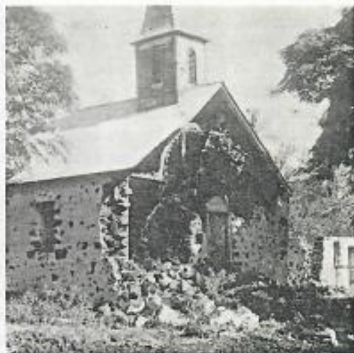
FIG. 7. Catholic Church 0.6 mile north of Hookena Beach, from the northwest. The east end of this church was similarly thrown down and outward, to the east. The near corner and the corresponding corner of the small building, already without a roof, suggest displacement most markedly to the northwest, in the general direction of the epicenter.
