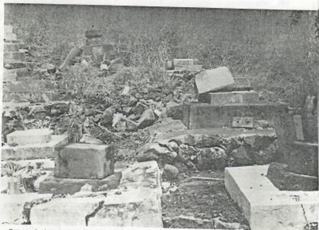
FIG. 11. Broken bases, displaced base stones, and overturned headstones in Kalahiki Japanese cemetery, south of Kealia, looking southeast. Partly because of unstable hillside ground and partly because of proximity to the epicenter, damage in this cemetery was widespread and severe; scarcely a grave escaped marked derangement.
