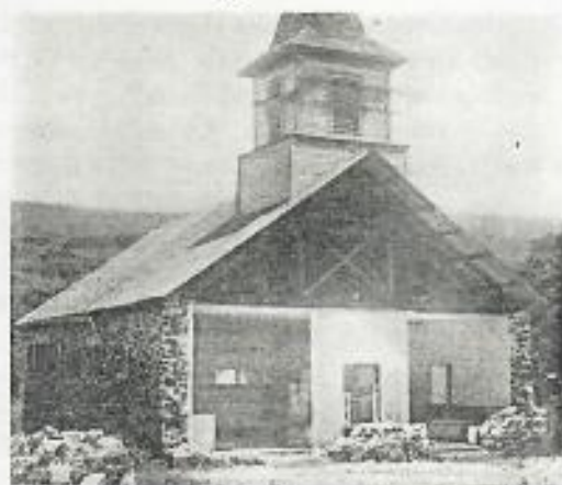
FIG. 6. West end of Pukaana Church at Hookena Beach showing complete demolition of masonry wall of this 100-year-old structure. Much of the debris was cleared away soon after the earthquake. No nearly comparable damage to this building is known to have taken place during the century since it was built.
