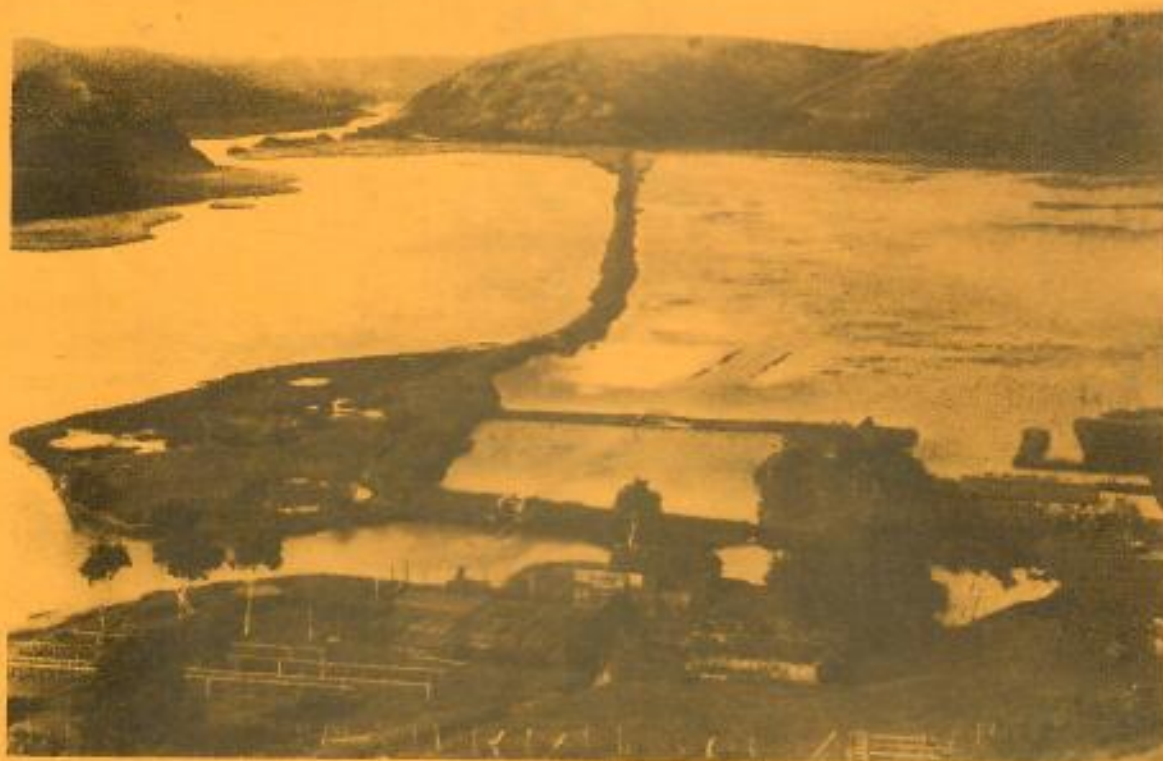
Alekoko Fishpond, circa 1930-40's, Hūleia. Details of secondary ponds, wall, structures and channel dug into the silted pond. Photo courtesy of the Kauai Museum, Neg PN 3030.14.
