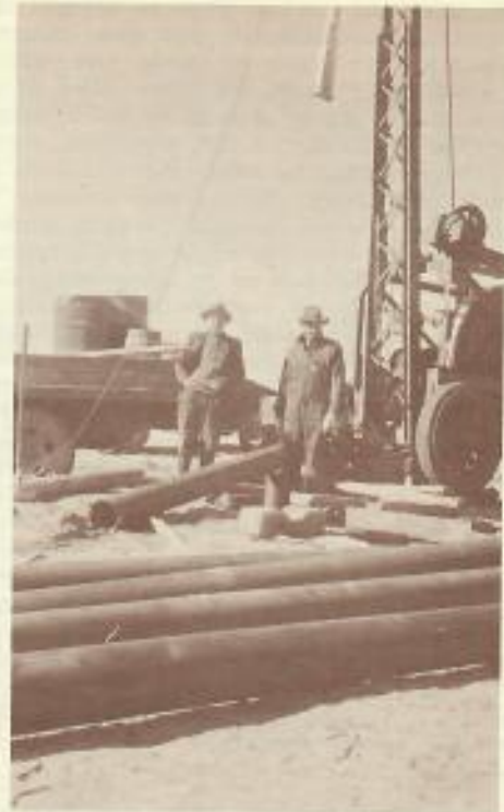
Edward Paxton and Mr. Stevenson, the well drifter - February 1939, bringing in one of the early wells on the Paxton acreage.
