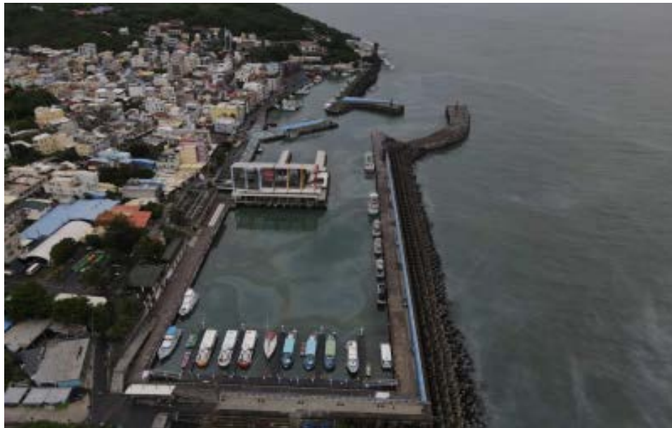
Dafu Wharf blackened by oil spill [credit: Su Huai]
