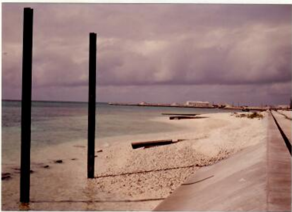
Plate 38.--Coral-rubble beach accreted along a 200-m portion of Johnston Island's south shore seawall, between the iron pilings (foreground) and the West Peninsula (seen in the distance).
