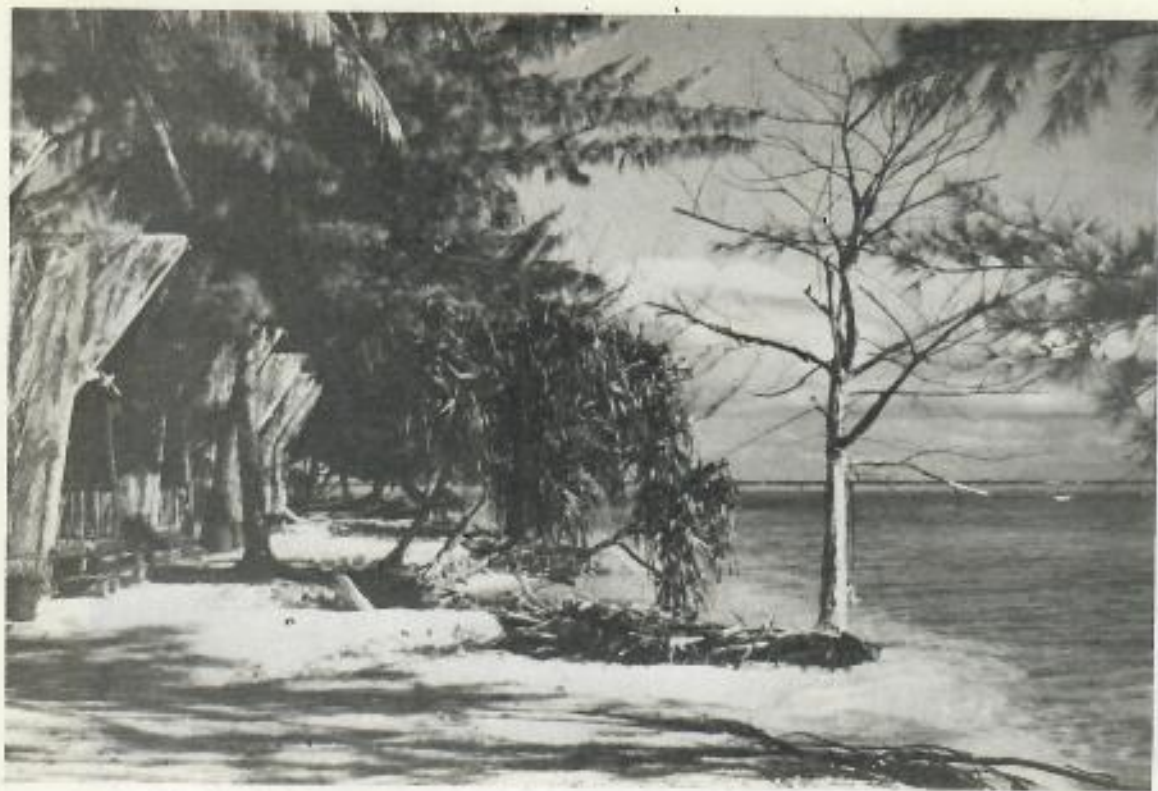
Fig. 37 Onetahi Islet, badly eroded beach front along passage; buildings were in use. MHS, 1982
