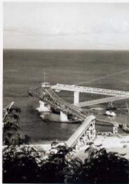
ABOVE / After phosphate was discovered on Makatea in 1906, it became a hub of a global mining industry. In the mid-1950s, a gigantic mobile gateway called "the grasshopper" (seen here) was constructed at Makatea's port of Temao to deliver ore directly from a train to cargo ships. PHOTO COURTESY OF LOUIS MOLEY / TAHITI HERITAGE
