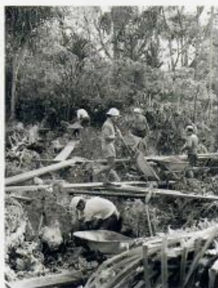
ABOVE / Dangerous excavations: Phosphate miners on Makatea in 1962 cart wheelbarrows loaded with phosphate sand along narrow footbridges spanning deep, limestone-walled pits. PHOTO COURTESY OF LOUIS MOLET / TAHITI HERITAGE
