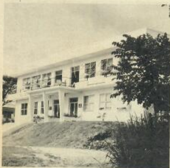
Above, the new Condominium offices, completed at a cost of $260,000, were opened towards the end of last year in true Condominium fashion—the two High Commissioners for the Pacific, French and British, cut a ribbon simultaneously. At the right of the Condominium office is part of the new store of Burns Philp (S.S.) Co. Ltd. The old store and office, which has occupied a quonset type building since the end of the war, is being pulled down. Left, the substantial-looking Vila Club, centre for local social activities.
