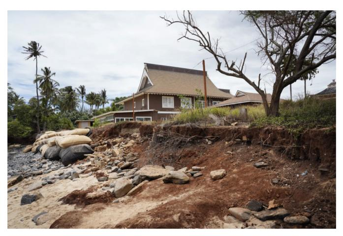
Sandbag revetments, also known as geotechnical containers, try to keep erosion at bay on the makai side of the Mantokuji Soto Mission. They are a temporary solution while the temple's board of directors and Oceanit try to figure out how to permanently protect the temple and associated graveyard from falling into the ocean. (Kevin Fujii/Civil Beat/2024)
