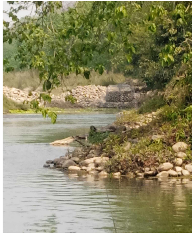
Figure 3. Gabion wall flanked by vegetation along bank of the Rapti River in CNP. Photograph: Bed Khadka.
