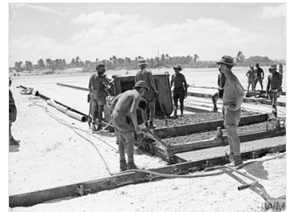
Royal Engineers construct the airfield runway.
