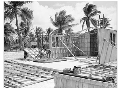
Royal Engineers assemble huts on Christmas Island
