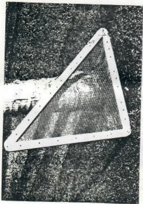
Figure 5. Triangular screen used on the outlet to the fish pen. Two screens were used, and consisted of galvanized wire bolted to a PVC plastic frame.
