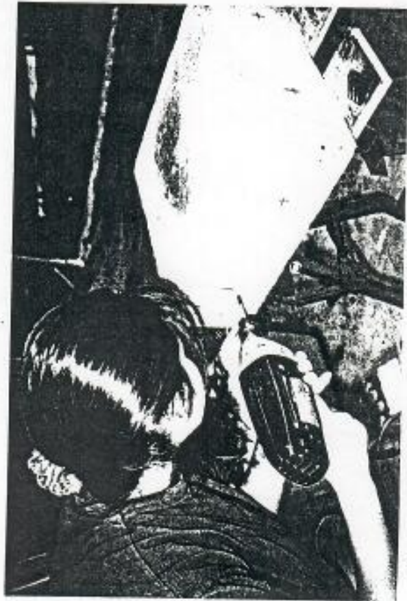
5. Drilling base for hardware
