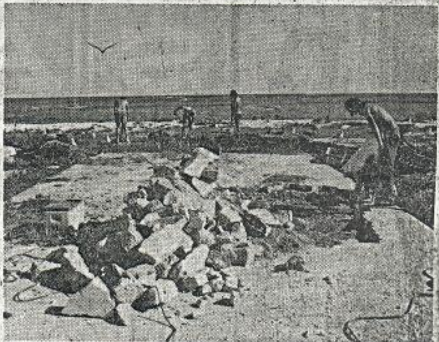
CLEANUP —Scientists break up the principal concrete foundation, measuring 20 by 65 feet, on East Island in order to make more space available for nesting by green sea turtles. —Photo by George H. Balazs.
