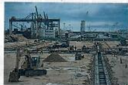
Construction at the Port of Guam , 2014
